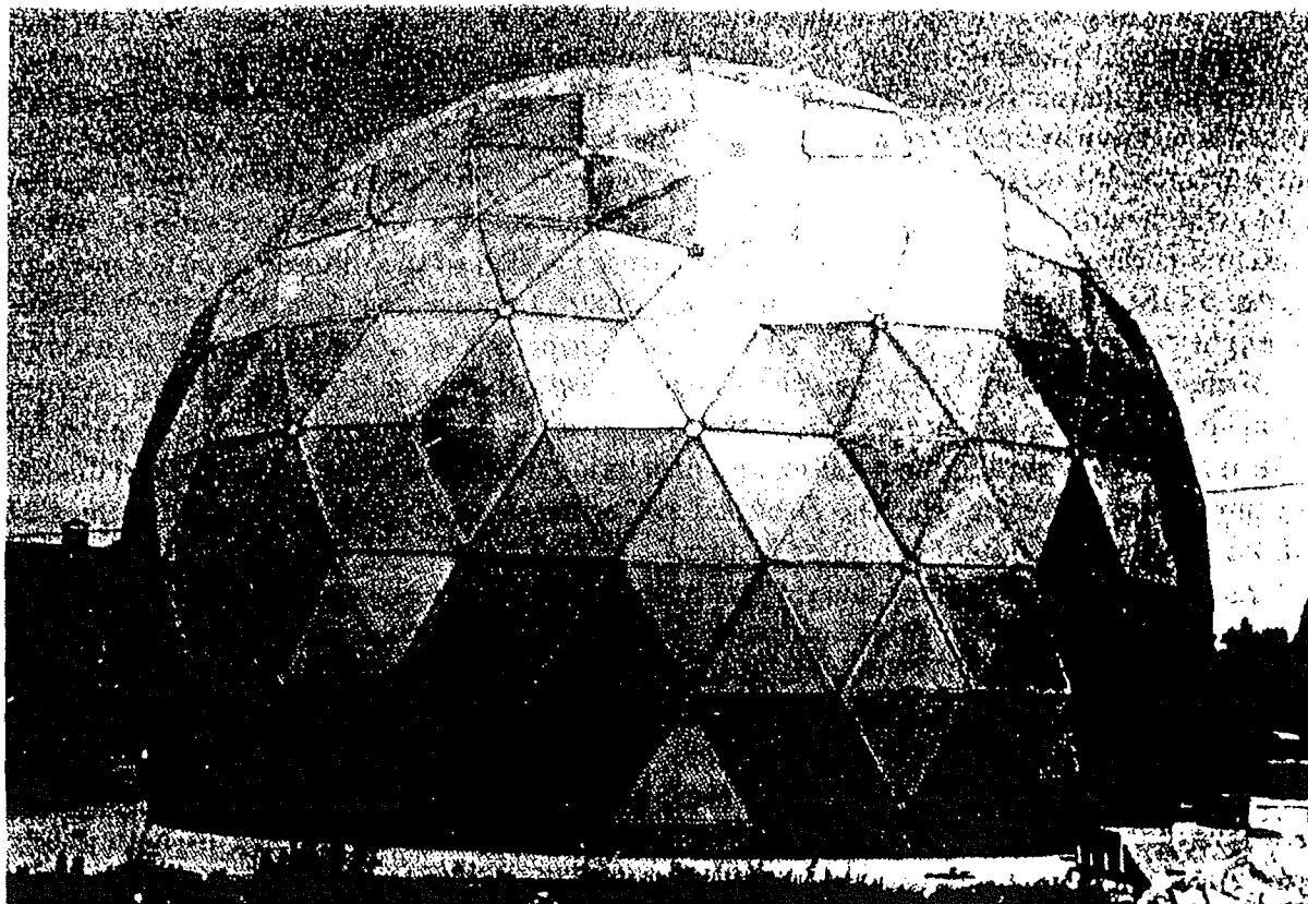
Figure 7.29 Rigid radome for ground-based antenna. (From Davis and Cohen, 125 courtesy Electronics and MIT Lincoln Laboratory.)
